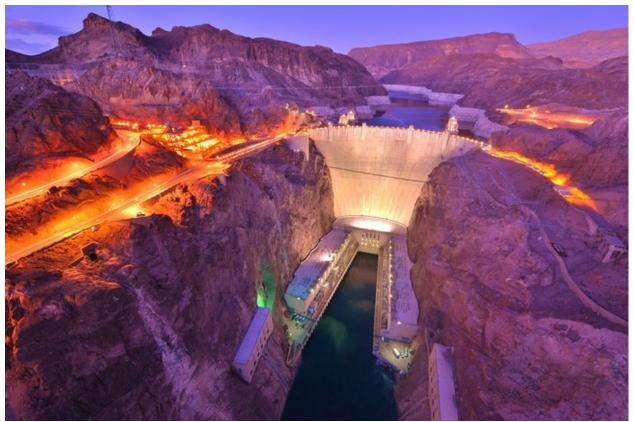
This dam is a concrete arch-gravity dam in the Black Canyon of the Colorado river, on the border between Nevada and Arizona
